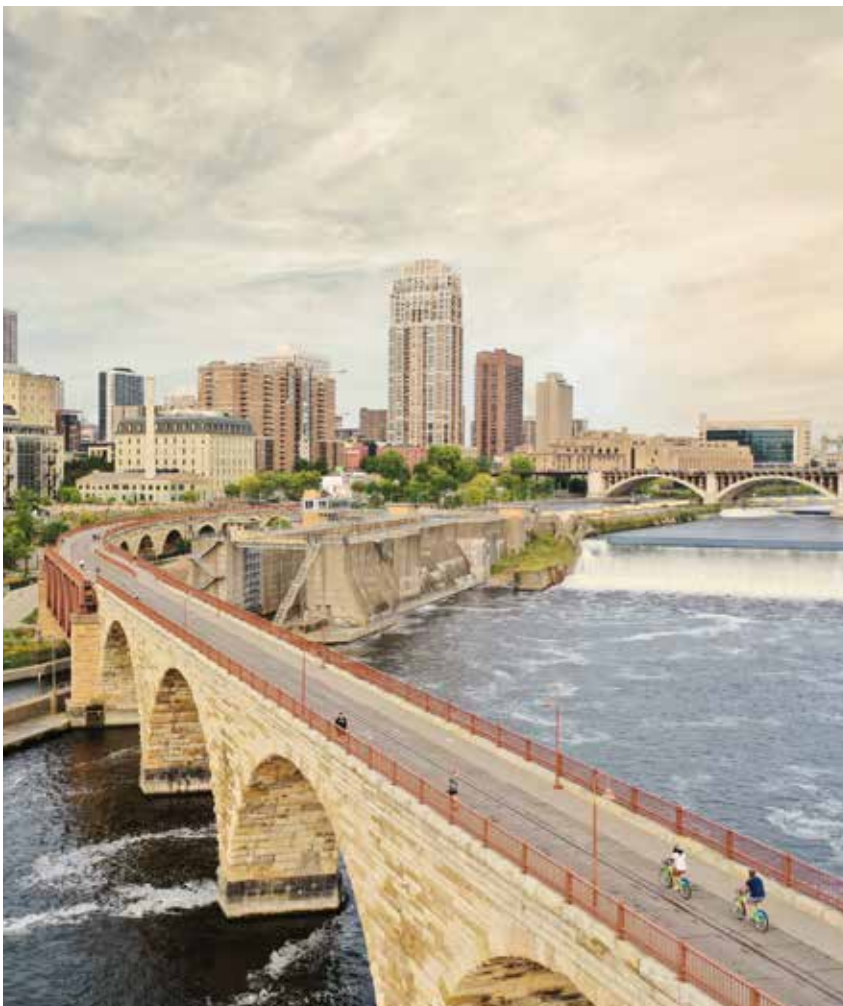
Minneapolis Stone Arch Bridge
